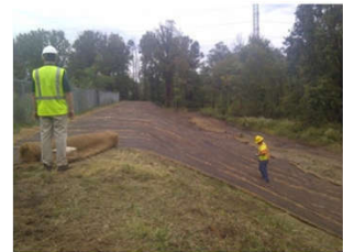
Reinforcement of impoundment berms in the south area.
