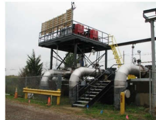
Elevated electrical controls for full-scale groundwater extraction.
