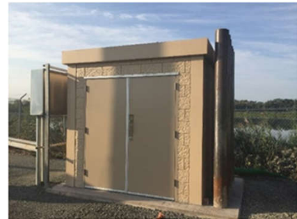
Onsite flood-resistant enclosure and bollards on concrete foundations.
